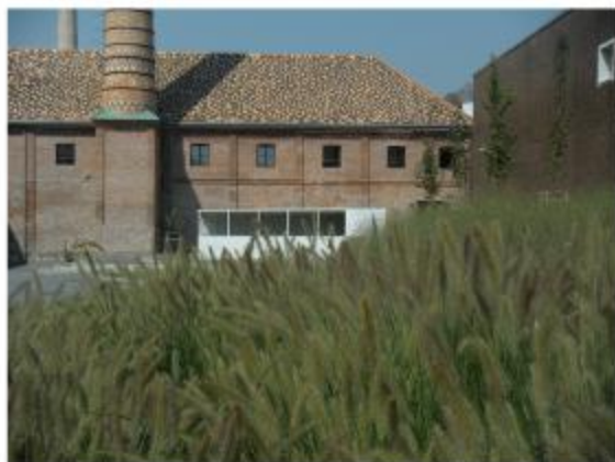
South pavilion / Büfö pavilion
