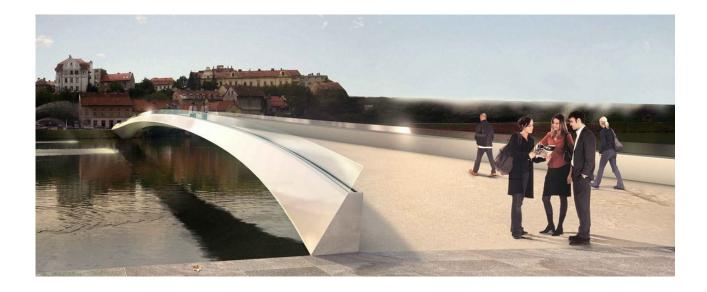
The jury was convinced by the structurally well elaborated and sound proposal, which includes all the relevant explanations regarding the structural integrity, stability, sustainability and durability. The structure avoids underground city infrastructure by pushing the construction site onto the riverbank.
