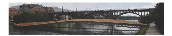
The surface rests on steel members cantilevering from a central spine built by two truss girders on two supports. It is very likely that the torsional stresses require additional members and will restrict the cantilever sizes. The project requires further refinements - structurally and in terms of geometry of the surface.
