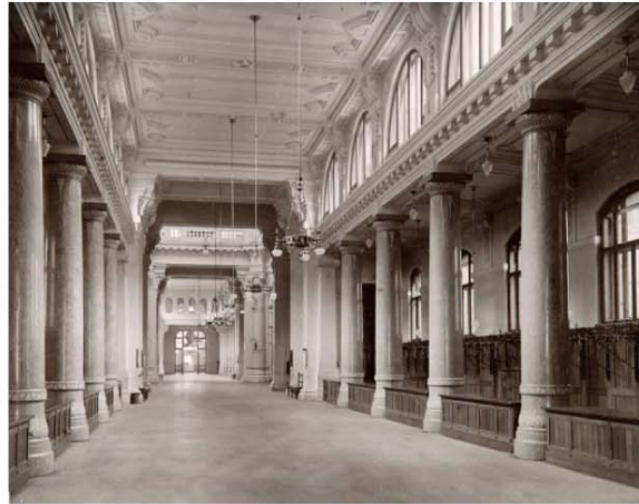
Northern Basilica Structure, 1908
